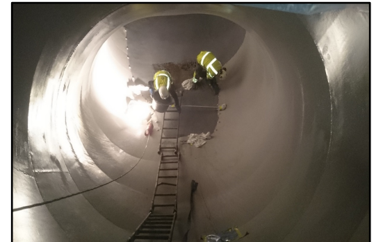
After: completing application of ARC 791
